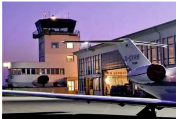
Tower Essen-Mühlheim (Germany)
