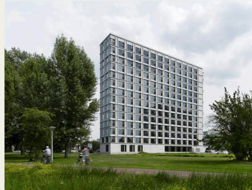
Student Housing Campus, Eindhoven BDG Architecten
