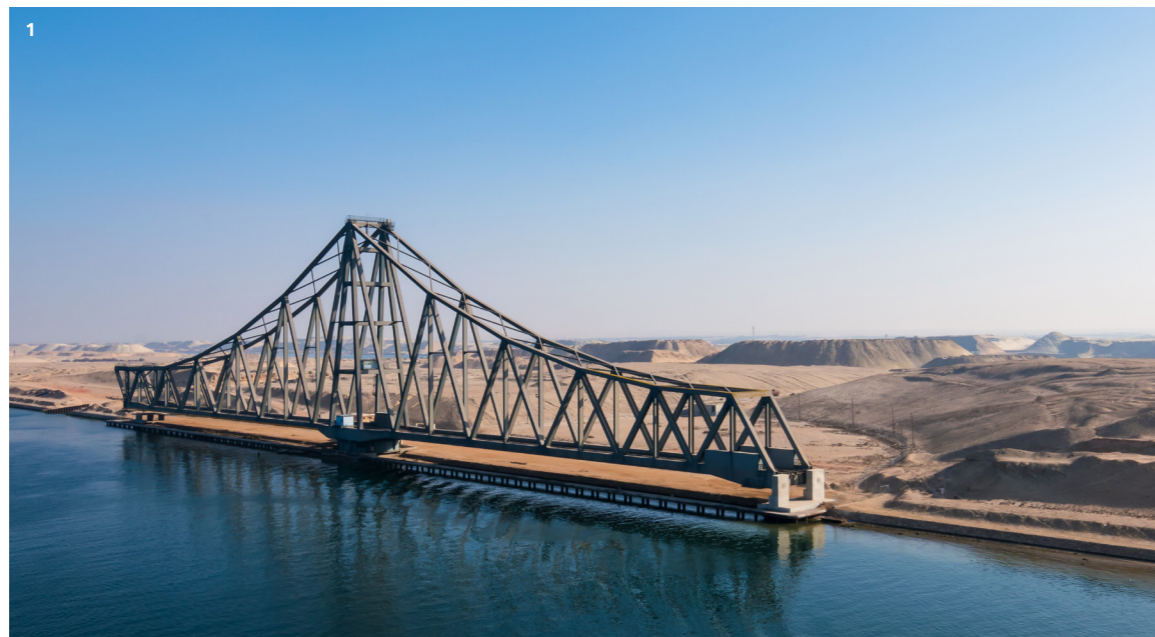
Figure 1 El Ferdan Railway Bridge, the longest swing bridge in the world, runs from the west of the Suez Canal to the east into Sinai, opens most of the time to allow sailing ships to pass in the canal.
