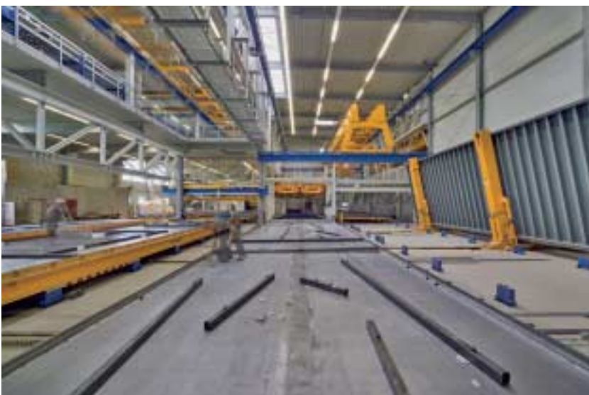
Fig. 12 In the demolding preparation area, the magnets of the shutterings are deactivated manually.
