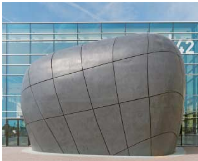
Fig. 2 The “Lake Constance Pebble” has been erected just recently. This building is a masterpiece not only in architectural terms but also from a manufacturing point of view.
