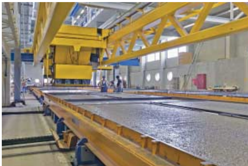
Fig. 7 The automatic concrete spreader is fitted with a spreading roller and discharge screws.
