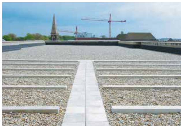
Abb. 24: Bekiestes Umkehrdach
