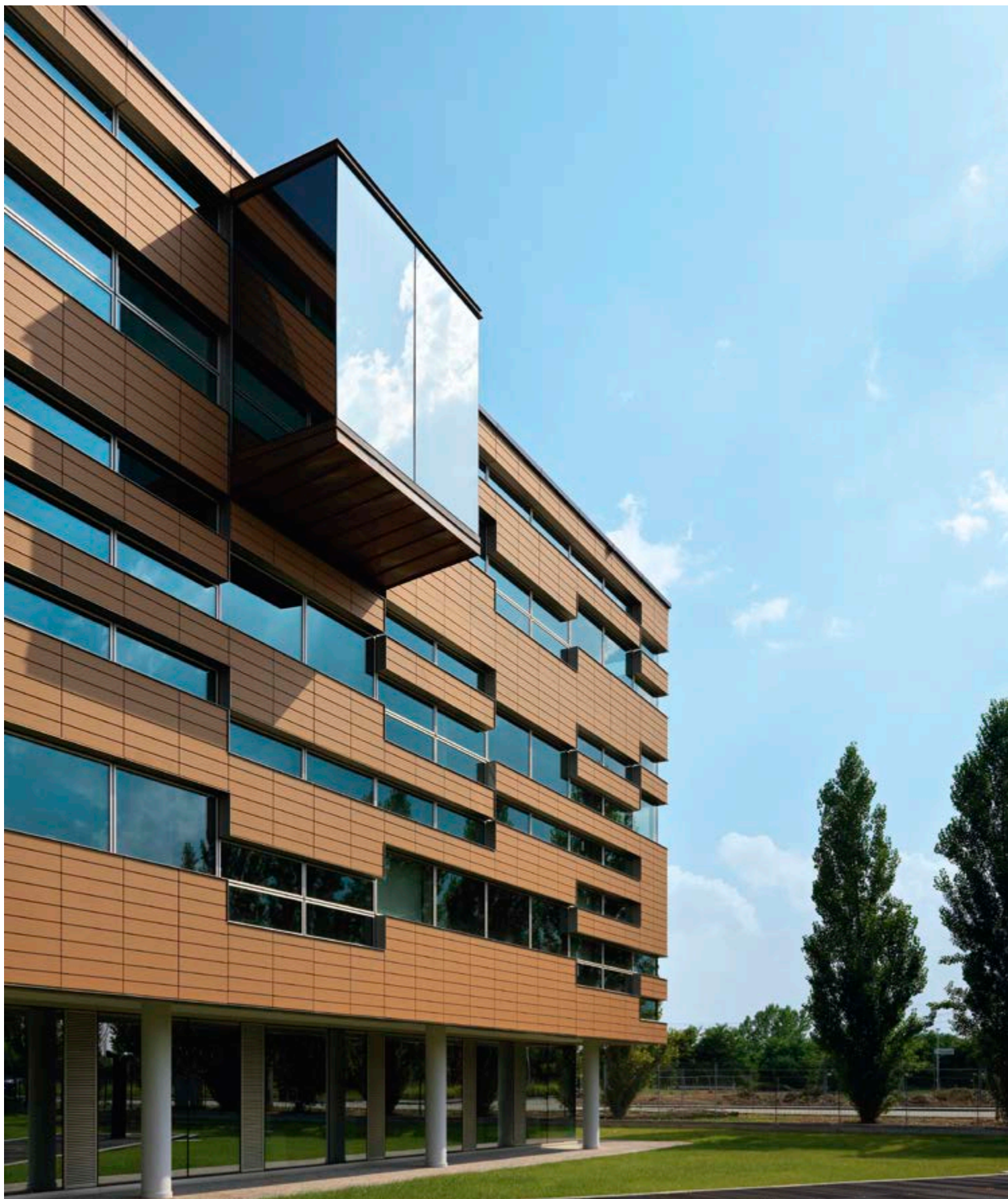
LEED PLATINUM Crédit Agricole Green Life Headquarter, Parma, Italien / Architekt: Frigerio Design Group/ Foto: Enrico Cano, Frigerio Design Group
