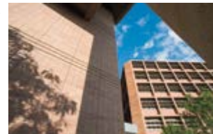
■ Lee Shan Building, Hong Kong, China
