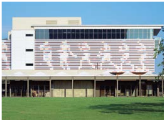
Muhammad Ali Center, Louisville, USA / Architekten: Lee H. Skolnick Architecture + Design Partnership
