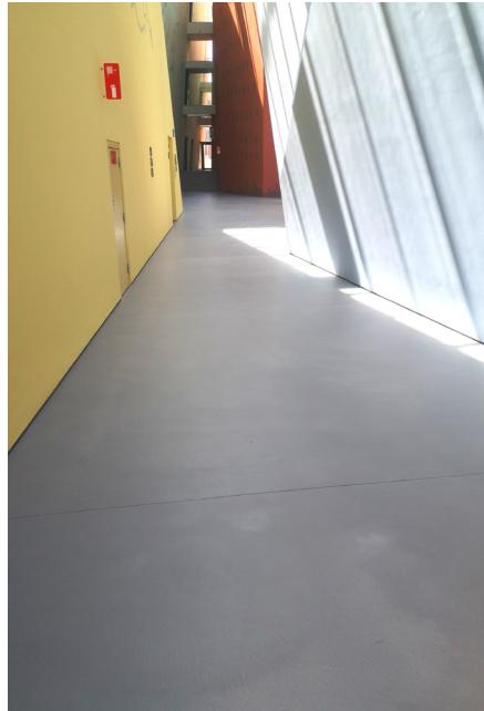
**EN** – Ideal Skin is a ready-to-use acrylic-based material which is extremely durable and easy to apply. It is also suitable for floors subject to heavy traffic and for use in bath and shower rooms. The Ideal Skin system includes special primers that allow it to be applied on most every solid substrate and background including screed, existing ceramic floor and plasterboard or plaster, as well as solid panels or furnishing accessories.
