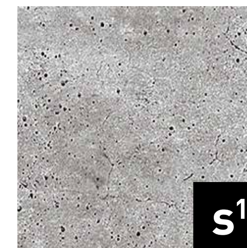
s1 beton concrete
