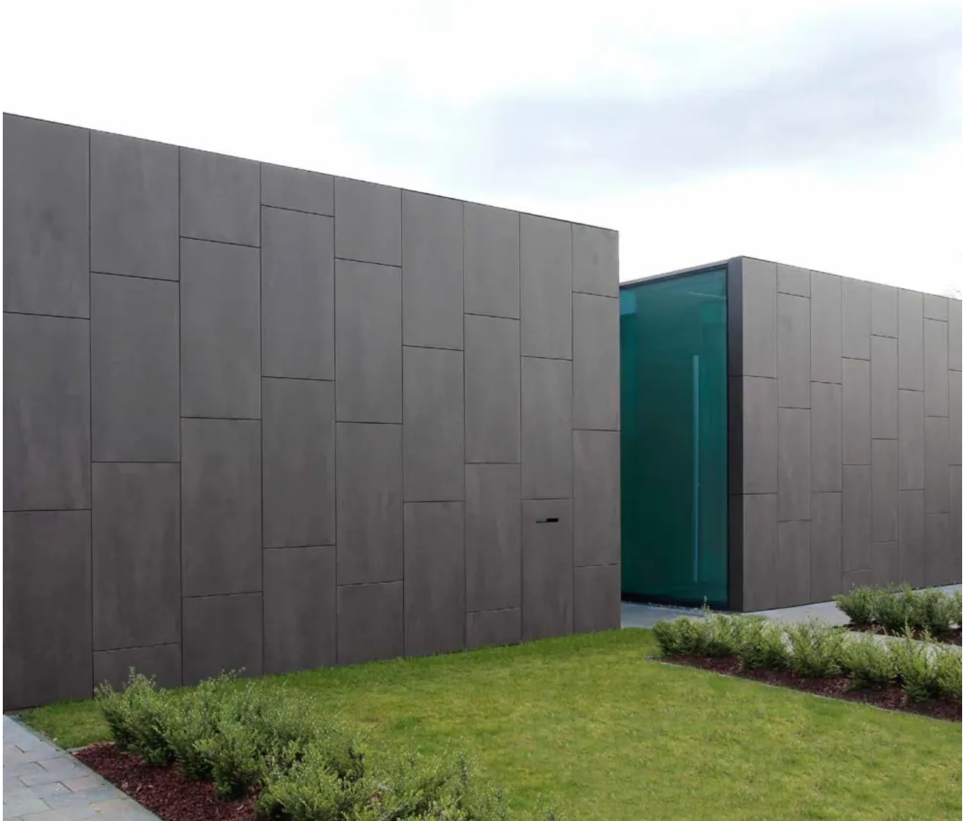
Faehuskervey private home Apeldoorn (NL) COURAGE Architects 2013 Terra Beige & Brown 265V
