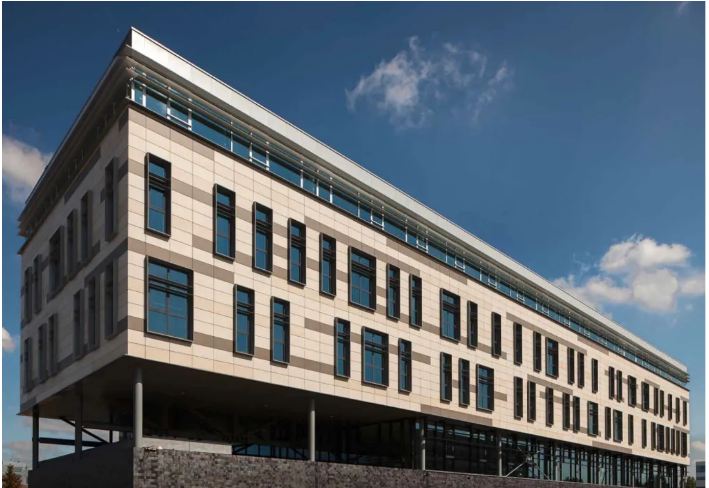
Blue Water Energy Services Hoofddorp (NL) N30 2014 Terra Maestricht 201V / 204V / 211V
